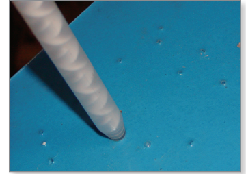
Figure 6: For short pot life urethanes, the material is simultaneously mixed and injected.
